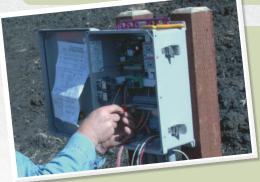
"I got a call from a contractor at 4:00 pm on a Friday (of course). He told me he'd hit the wires on a control panel and the alarm was going off. It was a 14-pump Orenco custom panel. He'd pulled the wiring right out of the terminal blocks, and one block was completely disconnected. The wiring to the logic controller was pulled out, too.
