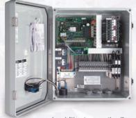
In addition to operating like other panels, the VeriComm Control Panel has four very "smart" functions: alarm management, data collection, troubleshooting, and advanced control logic. Operators can change settings at the panel from a PDA with Bluetooth®, or remotely via the web.
