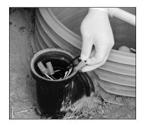
**WARNING:** Failure to use waterproof wire nuts can cause intermittent or permanent float failure.
