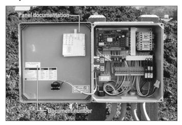
The system may have multiple control panels. Identify if there are control panels on the section of the system that you are about to start-up.
