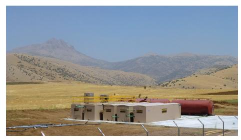
A seismic surveying firm needed portable wastewater systems for a series of remote camps in Iraq. The AX-Mobile was chosen for its ability to meet treatment limits with minimal operation and maintenance needs.
