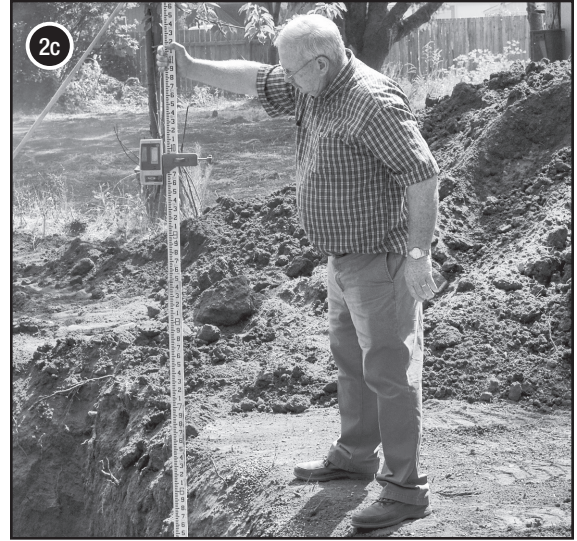
Make sure the excavation is stable, smooth, level, and free from debris, rocks, and sharp objects.
