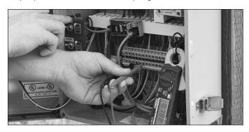
First for the recirculation pump and then for the discharge pump, measure the voltage with the pump off, by putting the probes of a voltmeter on each pump's terminals. Then measure the voltage with the pump running. The difference between running and rest voltage should be no more than
