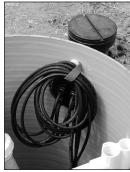
Splice box mounted in discharge access riser. Watertight connectors used.
