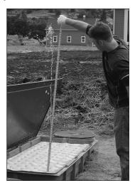
Inspect the discharge pump basin or tank to make sure that it is set level and there is no sign of water infiltration.
