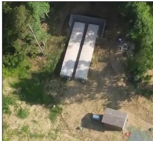
These AdvanTex AX-Max units are so easy to maintain that operator visits are only required every week – as opposed to the daily visits required for the old package plant.
