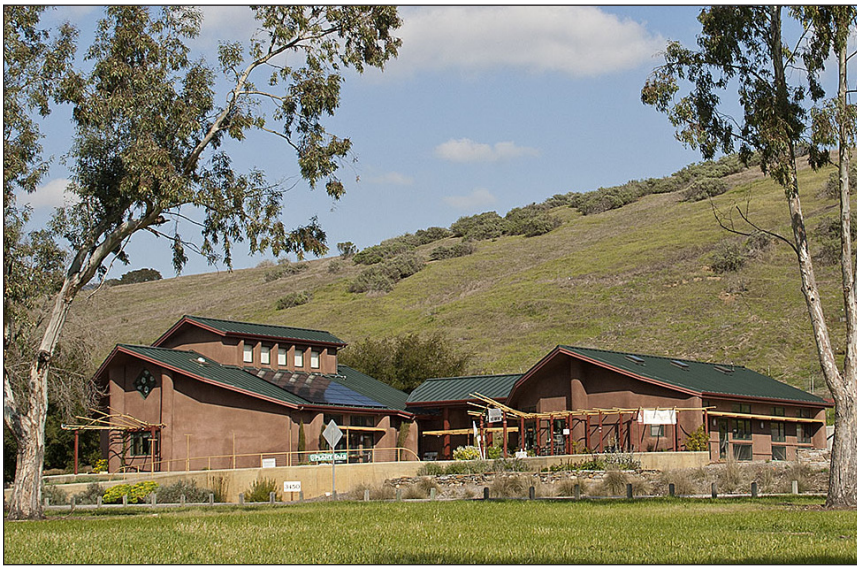
Two AdvanTex units with small footprints provide effluent that is reused for irrigation at the San Luis Obispo Botanical Garden. Photo courtesy of Ron Kindig, San Luis Obispo Botanical Garden.
