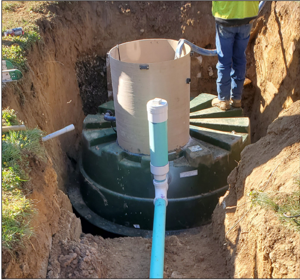
At the core of a Prelos Sewer is the Prelos Processor, featuring a long-lasting, lightweight effluent pump and a unique, patented "meander" design for superior solids settling, removal, and primary treatment.
