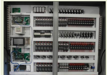
This TeleComm (TCOM)™ custom control panel installed at the Silverhorn community is a cost-effective, digital, integrated telemetry panel that features data logging, remote access, and control – all in real time.
