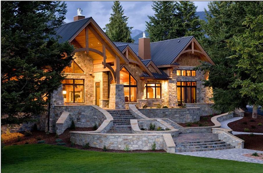
Silverhorn is a luxury community in a country setting. The development's wastewater is treated by four AdvanTex® AX100 Treatment Systems, operated through a custom TCOM™ control panel by Orenco Controls™. Photo courtesy of Silverhorn Inc.
