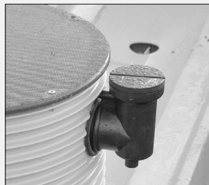
External splice box installed on riser.
