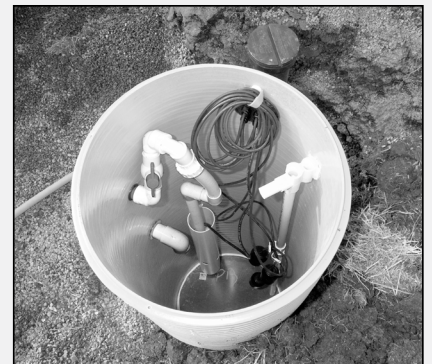
Interior of a finished pump basin.
