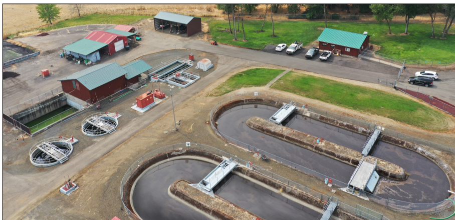
Liquid-only sewers operate under pressure and are tested for watertightness, so they're typically free of infiltration, which translates to a lower hydraulic load at the treatment facility.
