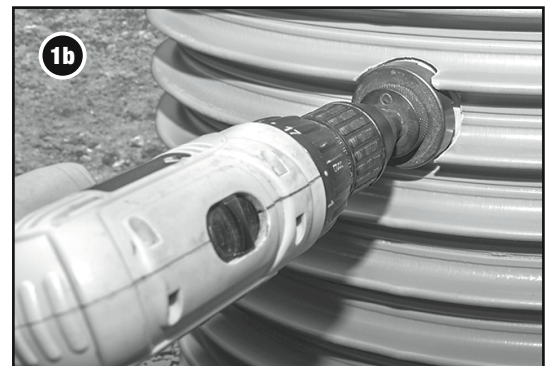
Drill the splice box hole.
