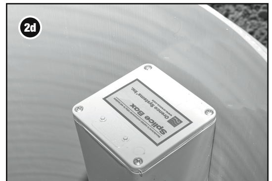
Install splice box.
