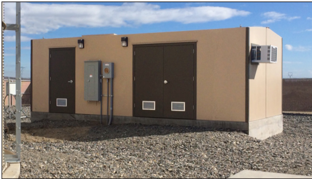
This DuraFiber utility building at the Love's Travel Stop is made of a fiber-reinforced polymer that's superior for many commercial applications. Vacuum-infusion molding makes the building exceptionally strong.
