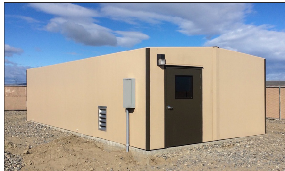
The travel stop also has a larger DuraFiber building that houses pumping equipment and chemicals for the wastewater system. Like the water utility building, it came with interior and exterior lighting, heating, ventilation, and air conditioning.
