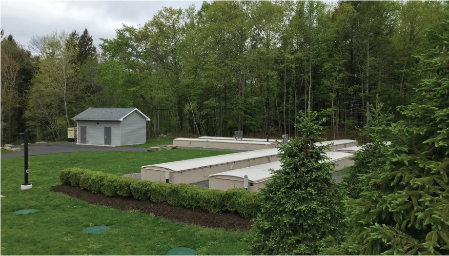
An AdvanTex AX-Max Wastewater Treatment System – with its low life-cycle costs and small footprint – was chosen as the best replacement for a failing treatment plant in the community of Pinebrook, New York. Photo courtesy of Julie Barown.
