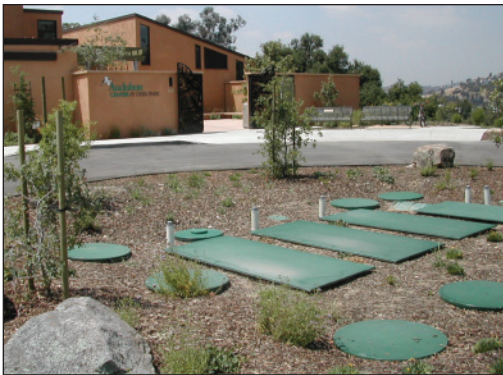
The Audubon Center's AdvanTex Treatment System produces such high-quality effluent that it is reused for irrigation, and, when permitted, will also be reused for toilet flushing. Photo courtesy of BioSolutions, Inc. ©2004.
