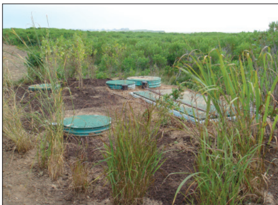
An AdvanTex® Treatment System, manufactured by Orenco, nestles discreetly in the beach grass. This low-energy, highly reliable media filter replaced the former cesspool and treats this Esther's Island household's wastewater to reuse quality. Photo courtesy of Scout Capital.
