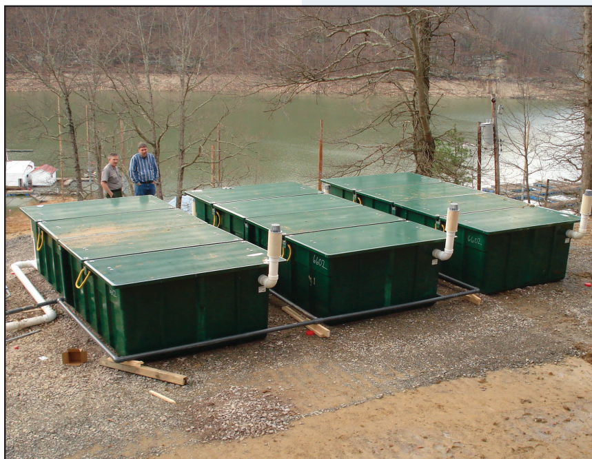
The AdvanTex pods were installed directly on top of the sand filter site.
