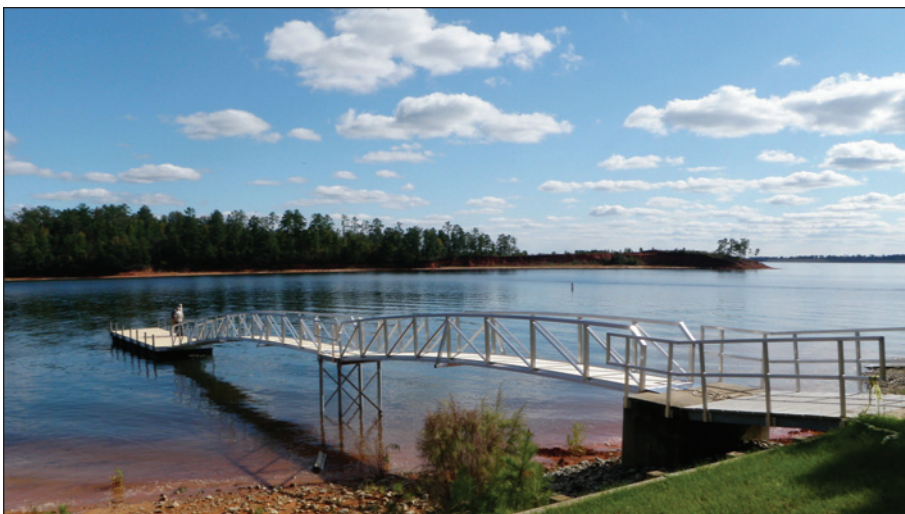
The U.S. Army Corps of Engineers was under time pressure to replace a wastewater treatment facility on Lake Thurmond.
