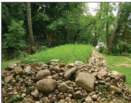
The existing drainfield on the east side of the house was replaced with a small, 300 sq ft box mound dispersal area.
