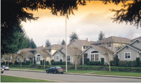
Developing efficient maintenance protocols has helped Lacey operate its hybrid sewer system economically.
