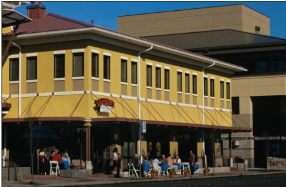
Lacey, Washington has a hybrid wastewater system with about 100 miles of gravity sewer lines (11,500 connections) and about 50 miles of effluent sewer lines (3,758 connections).
