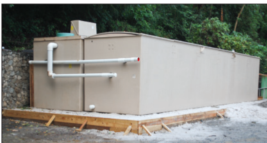
The resort needed two AX-Mobile units — one for tankage and one for treatment — to meet its emergency wastewater needs, and has since added a second treatment unit. These will become part of the resort's permanent wastewater solution, after equipment from the ruined system is removed.
