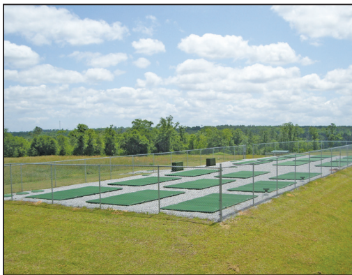
Phase I and Phase II of SAU's West Mobile wastewater treatment facility includes 36 AdvanTex AX100 textile treatment units. Two additional phases of similar size are planned. Another 18-pod textile treatment system is under construction in a different location.
