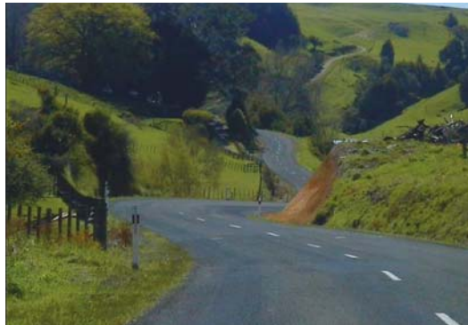
With an effluent sewer system, shallowly-buried collection lines follow the contour of the land, making them relatively easy to install despite the hilly terrain around Piopio.
