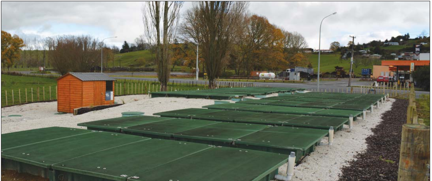
Located on the edge of the township, the fifteen AX-100 units in Piopio's wastewater treatment system draw little attention, as they are low-profile and emit minimal noise or odor. These low-maintenance units can also be installed further above ground, if desired.
