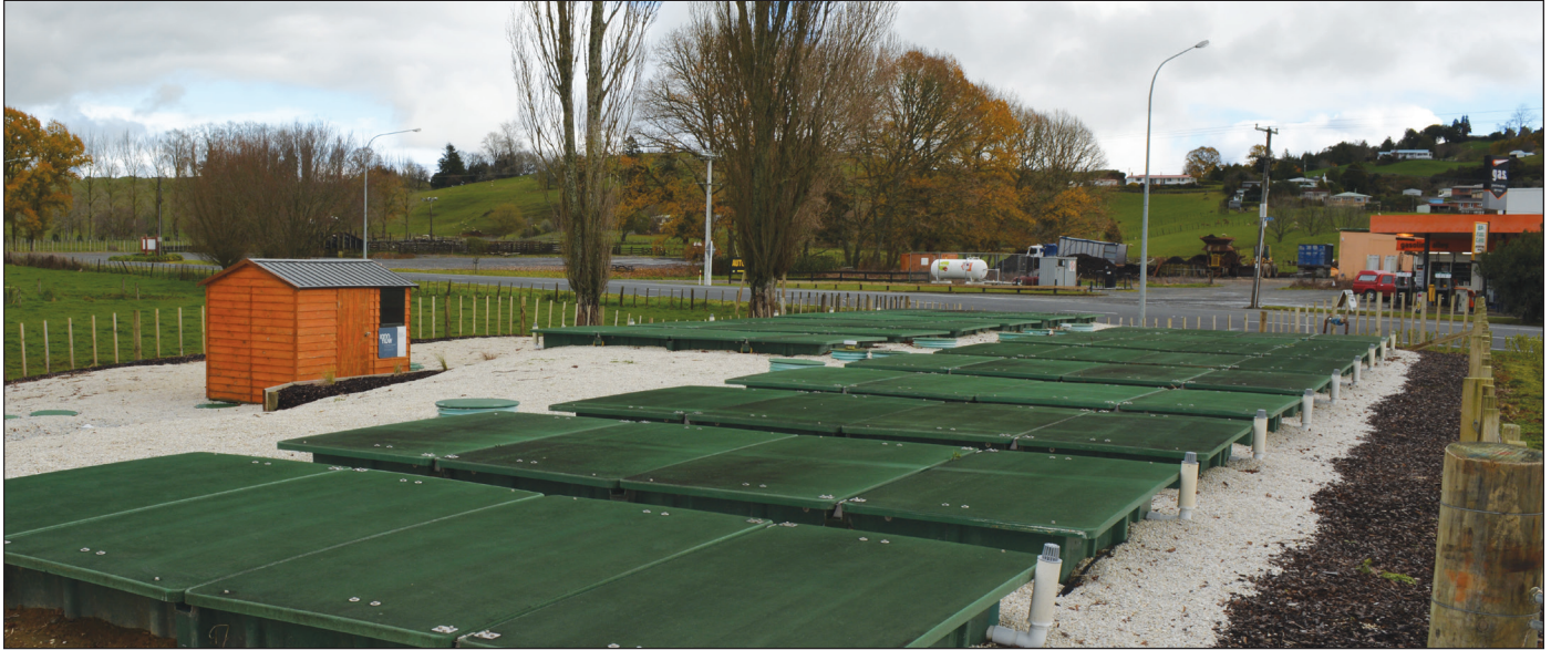
Located on the edge of the township, the fifteen AX100 units in Piopio's wastewater treatment system draw little attention, as they are low-profile and produce minimal noise or odor. These low-maintenance units can also be installed further above ground, if desired. Photo courtesy of InnoFlow Technologies.
