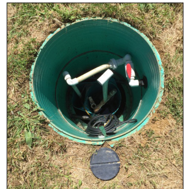
The Orenco high-head effluent pump housed in the pump vault has a life expectancy of over twenty years.
