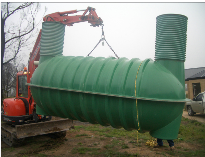
Undigested solids accumulate slowly in the on-lot tank, so pump-outs are typically needed only once every ten years.
