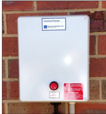
A control panel at each home monitors the components of the on-lot STEP package.
