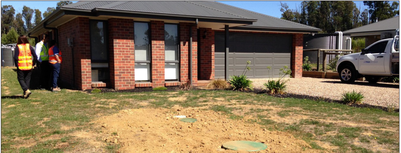
Each home received an Orenco STEP package, which includes a buried, watertight tank. Naturally occurring bacteria in the on-lot tank passively digest organic solids, making it possible to significantly reduce the size and cost of the treatment facility.
