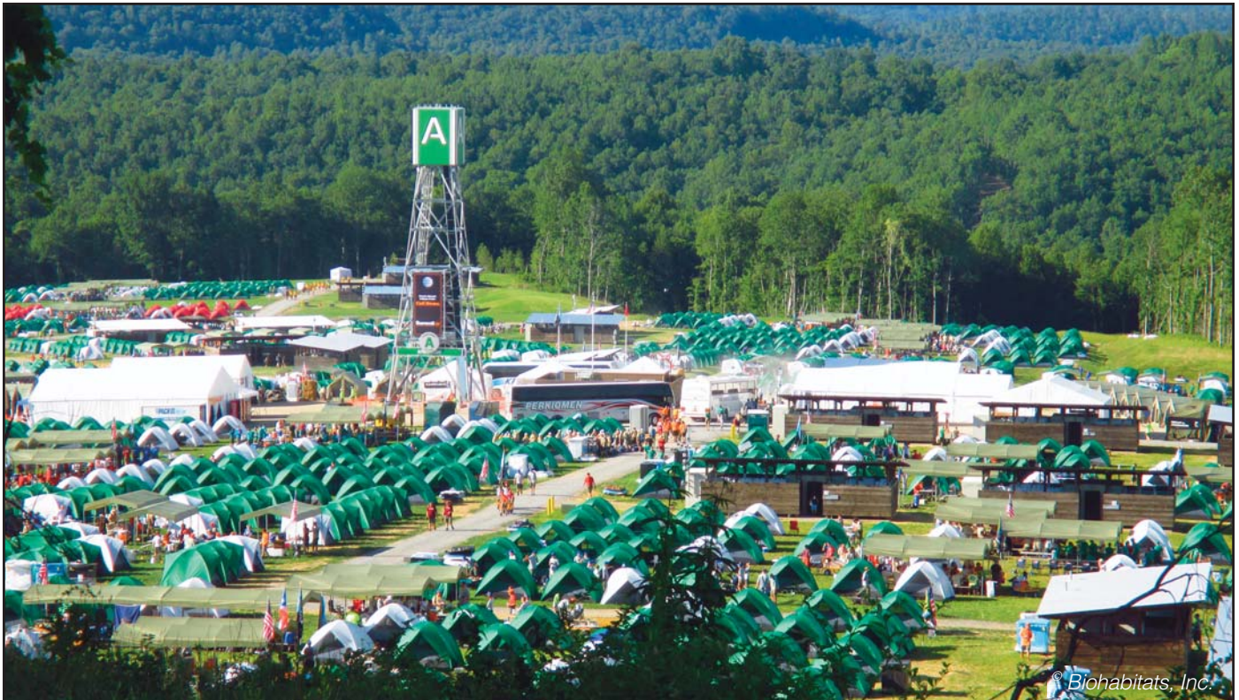
The AdvanTex Greywater Treatment Systems in place at the Summit Bechtel Reserve are an important part of the facility's overall sustainability. AdvanTex technology is known for its low energy use and for effective treatment, even with the highly variable flows common to camping areas.
