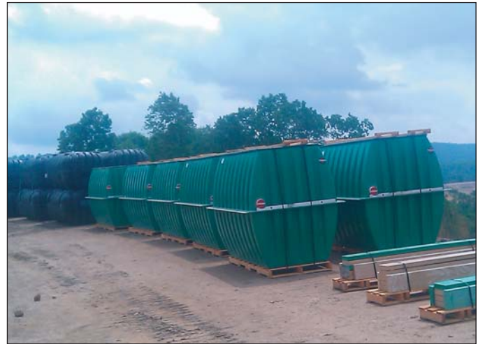
Engineers recommended these AdvanTex AX20-RT units due to the many advantages they offered, including a small footprint and a proven performance record for greywater treatment.
