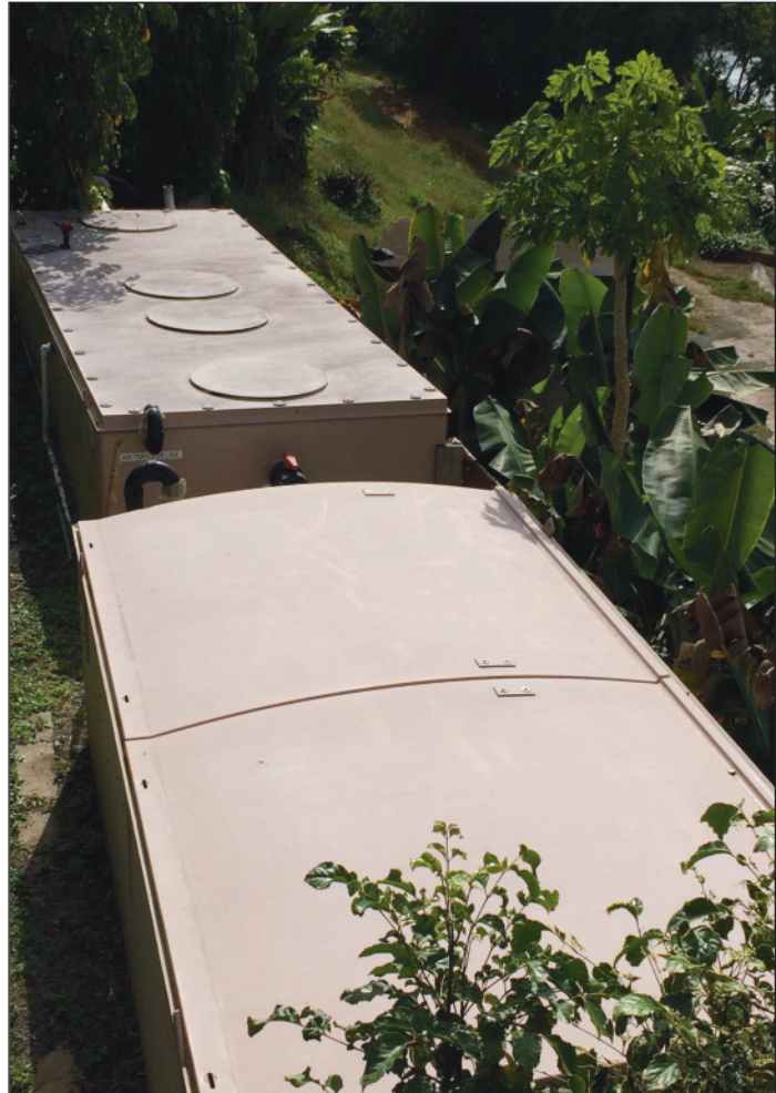
The Mountain Top condos use a T-Max™ tank for primary treatment, followed by a 4.3-meter (14-ft) AdvanTex AX-Max™ Treatment System. Together, they handle up to 11.4 m 3 /day (3,000 gpd).
