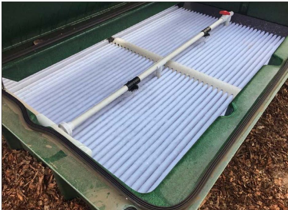
Treatment media in the AdvanTex AX100 is a uniform, engineered textile, which is readily serviceable and allows significantly higher loading rates than traditional recirculating gravel or sand filters.
