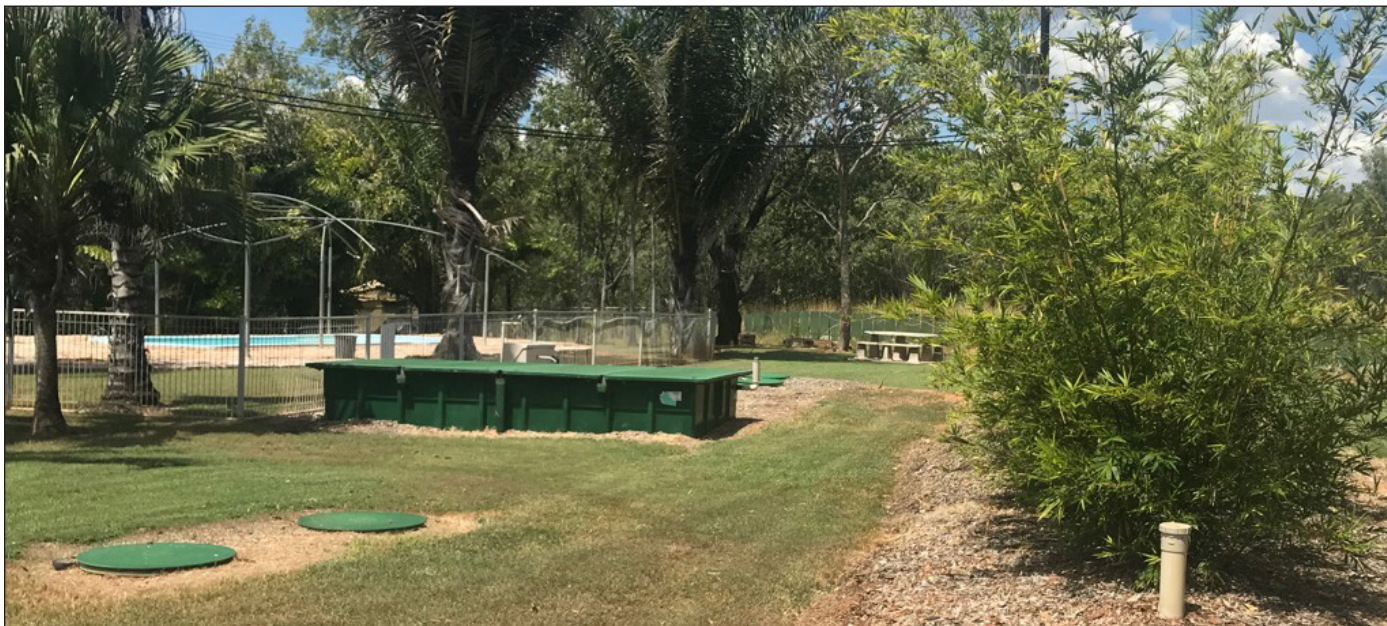
The AdvanTex system provides high-quality secondary wastewater treatment. Treated effluent is then dispersed through an ENVIRA Integrated Transpiration System, consisting of evapotranspiration beds (on the right) planted with select vegetation. Photo courtesy of ENVIRA Holdings.
