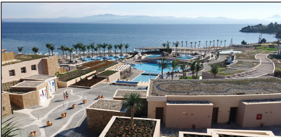
An AdvanTex® Treatment System handles up to 240 m 3 /day (63,400 gpd) of wastewater at the Miraggio Thermal Spa Resort in Greece. The effluent meets strict quality standards, and the system can be expanded to allow for future growth at the resort.
