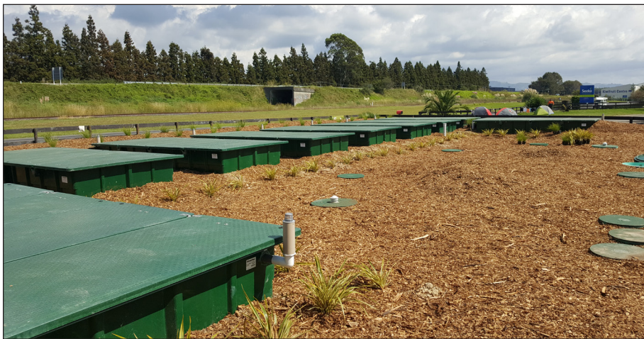
Installation and start-up of the AdvanTex treatment facility took place in only six weeks – in time for the start of the harvest and packing season that would bring an influx of seasonal workers.
