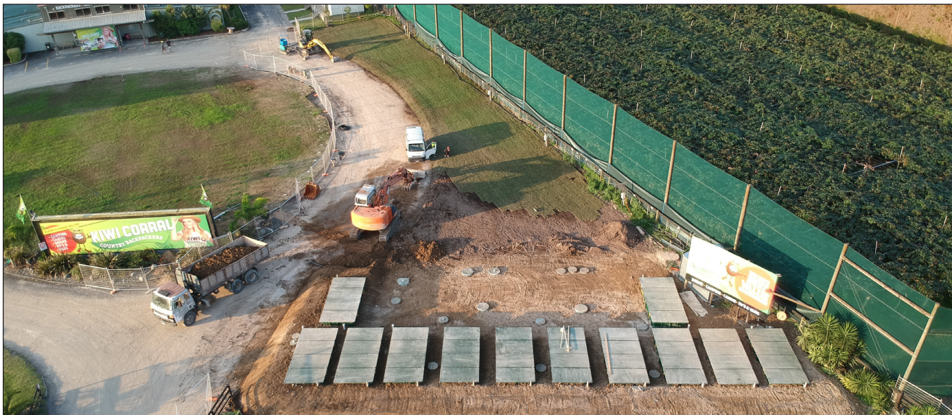
Construction plans were constrained by the size of the site: a space of only about 15 by 25 meters (49 by 82 feet). To reduce the facility's footprint, large process tanks were built on-site, and the AdvanTex treatment units were then positioned on top of them.
