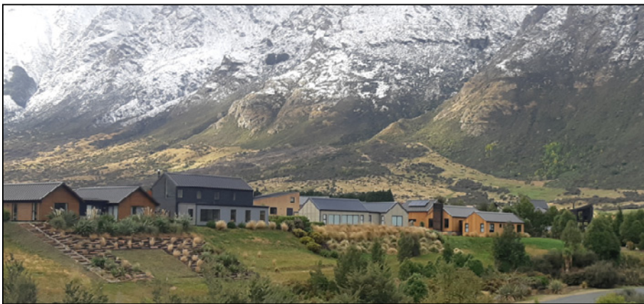
The developers of Jack's Point envisioned a subdivision of 900 luxury homes. They needed an affordable wastewater collection system that could handle variable terrain, followed by a reliable treatment system that would produce high-quality effluent and could be installed in stages.
