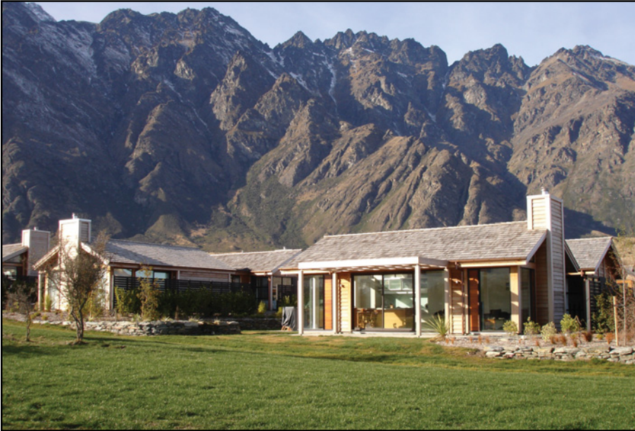
Using a liquid-only sewer at Jack's Point has reduced upfront capital expenses, because on-lot tanks are installed only as each home is built. Photo courtesy of InnoFlow Technologies.
