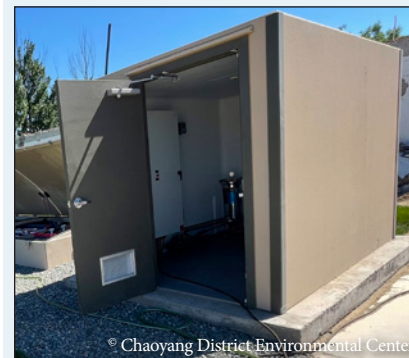
A DuraFiber building by Orenco Composites is also part of the facility and securely houses the TCOM control panel.
