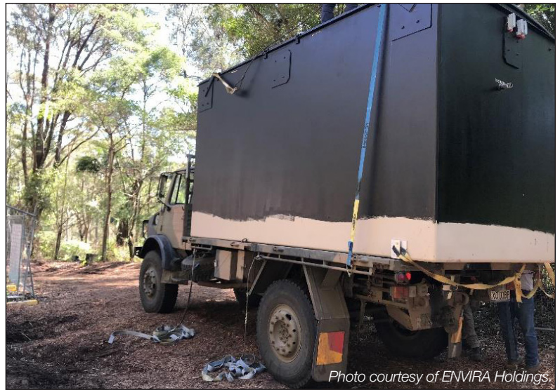
Photo courtesy of ENVIRA Holdings. The versatility of the AX-Max design allowed it to be split into two units per site, so that each unit could be transported up the mountain via truck. To blend in more fully with the environment, each unit received a custom paint job.
