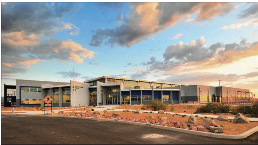
Orenco's AdvanTex Wastewater Treatment System was installed at the Andrada Polytechnic/Pantano High School campus near Tucson. (See story on reverse.)
