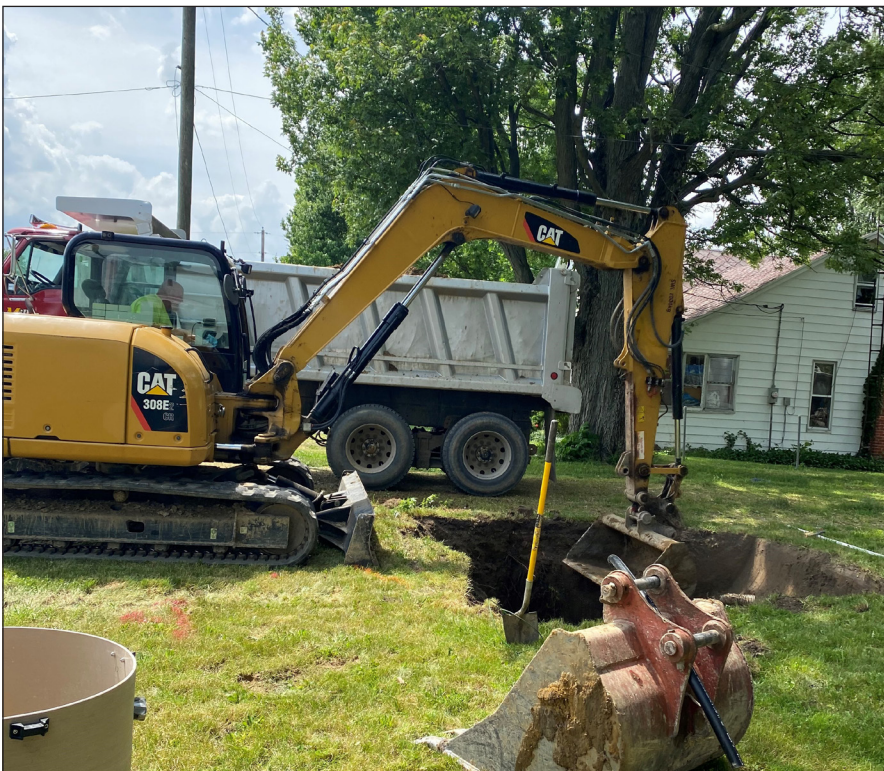
In a Prelos Sewer, a Processor is installed underground at each home. Small-diameter service lines carry the primary-treated effluent from the Processor to the AdvanTex treatment facility.
