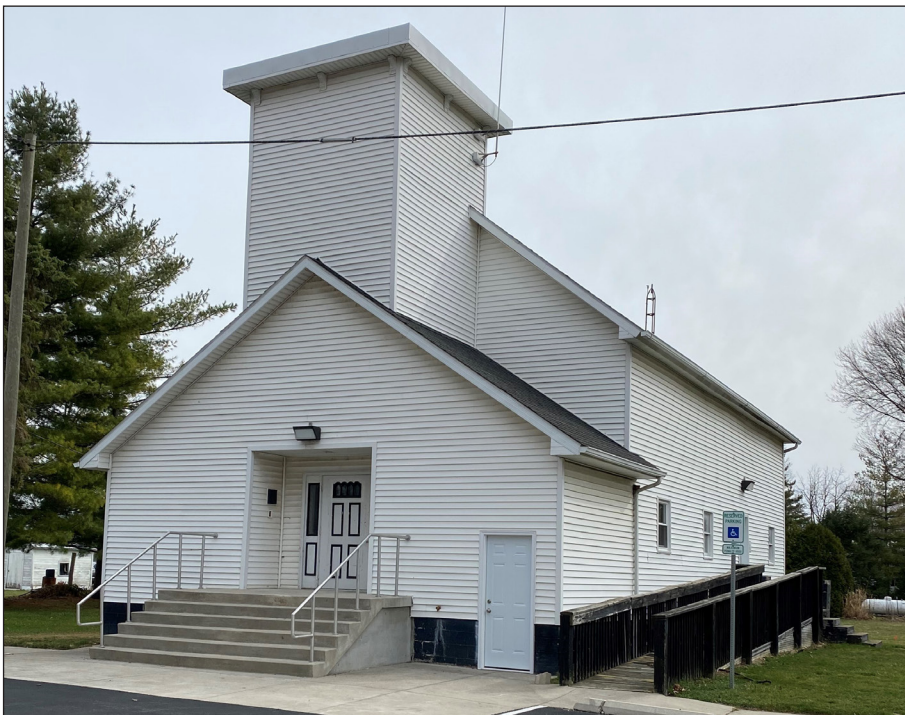
The villages of Dupont and Cloverdale joined forces to obtain funding from the Ohio EPA for their new Prelos Sewer and AdvanTex Wastewater Treatment System, which now allow them to discharge into the Auglaize River without polluting it.
