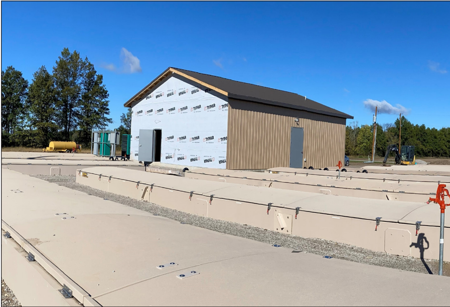
Construction crews bored underneath the Auglaize River to install the small-diameter sewer pipes that connected each village to this shared AdvanTex treatment facility. AdvanTex is an excellent solution for small communities and small-flow applications.
