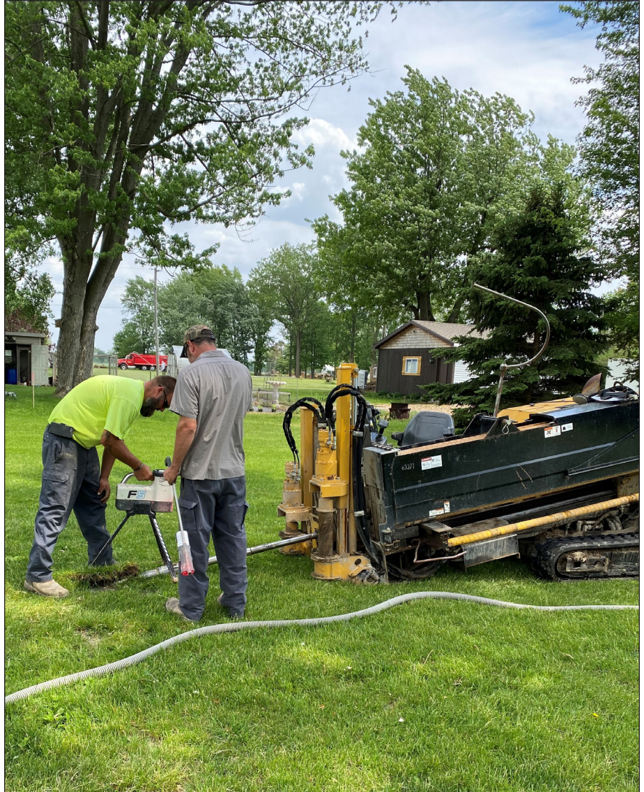
Trenchless construction is a less intrusive method of installing the small-diameter service lines used in a Prelos Sewer. It helps reduce environmental impacts and neighborhood disruption.
