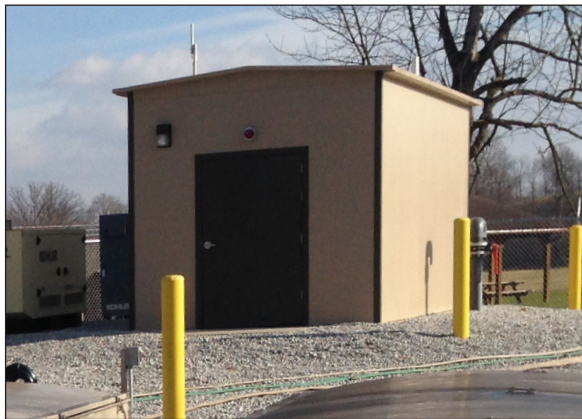
Manufactured by Orenco Composites, this DuraFiber building houses an Orenco Controls TCOM™ panel that provides monitoring and control for the wastewater treatment facility.
