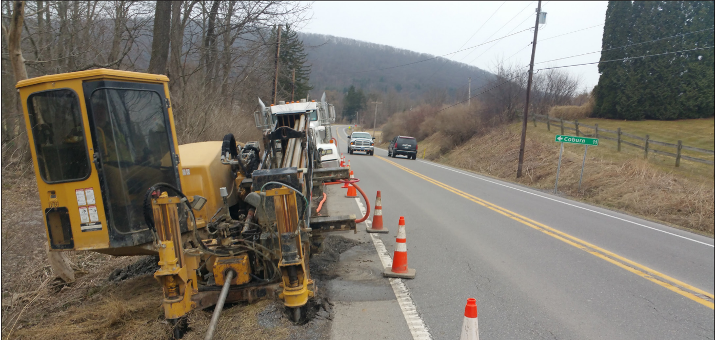
A Prelos Wastewater Collection System allows sewer lines to be installed using horizontal directional drilling, minimizing disruption to the community.
