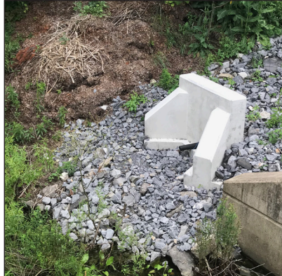
Treated effluent is pure enough to be discharged into a nearby creek.
