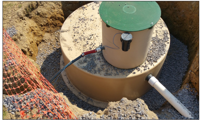
The Prelos Processor includes a patented "meander" design for superior solids settling, along with a patent-pending, passively self-cleaning pump vault, and a lightweight, low-horsepower effluent pump.
