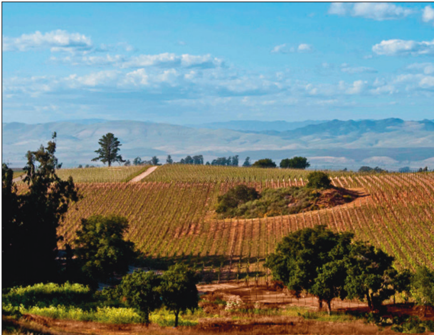
Summit Engineering, Integrated Water Services, and Cello & Maudru Construction teamed up to install six of Orenco's AdvanTex ® AX100 treatment units at the Presqu'ile Winery. Photo: Presqu'ile Winery, Santa Maria, California.
