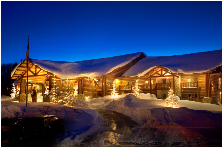
Daniels Summit Lodge in Utah, attracts outdoor enthusiasts year-round. This beautiful mountain location installed an AdvanTex wastewater treatment system to accommodate a restaurant expansion. Photo courtesy of Daniels Summit Lodge.
