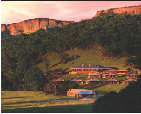
Emirates Wolgan Valley Resort and Spa, an eco-resort in Australia, chose a low-impact AdvanTex system for its environmentally sensitive site. Effluent is disinfected and used for irrigation.
