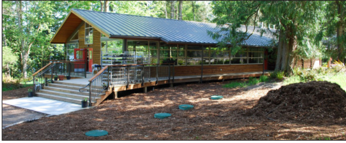
The refurbishment of Camp Fircom featured not only a new AdvanTex wastewater system, but also a dining hall designed by Principle Architecture. Photo courtesy of Camp Fircom.
