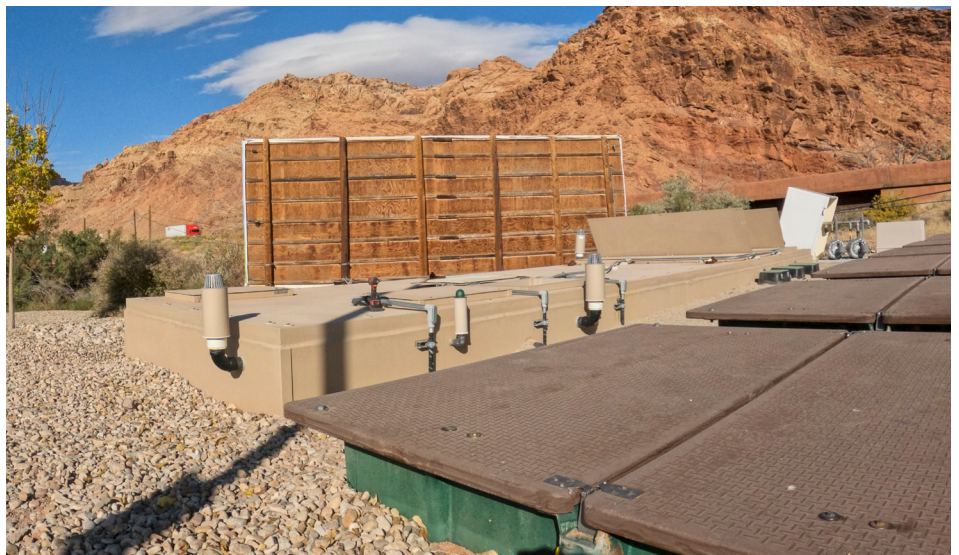
OmniMax-A uses aeration and biofilm media in motion to maximize contact, efficiently breaking down pollutants and reducing activated sludge.
