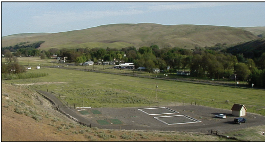
Aerial view of Starbuck, Washington, and its AdvanTex Treatment System.
