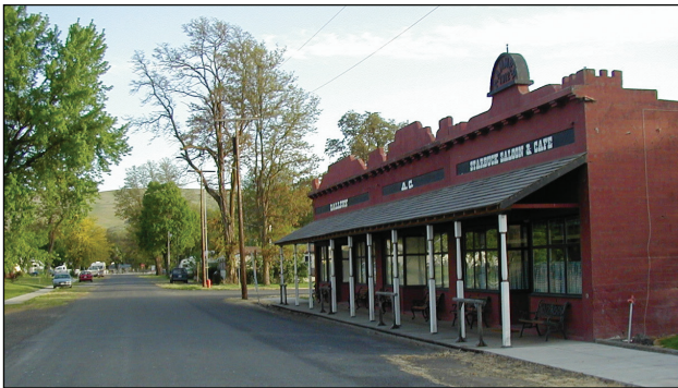
The small eastern Washington town of Starbuck (pop. 165) installed a low-cost, reliable effluent sewer system to serve the community, followed by an AdvanTex Treatment System.
