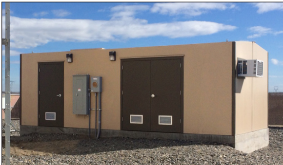
This DuraFiber™ water utility building at the Love's Travel Stop is made of a fiberglass-reinforced polymer that's superior for many commercial applications. Vacuum-infusion molding makes the building exceptionally strong.
