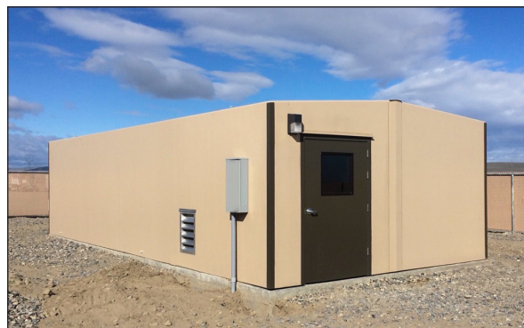
The travel stop also has a larger DuraFiber building that houses pumping equipment and chemicals for the wastewater system. Like the water utility building, it came with interior and exterior lighting, heating, ventilation, and air conditioning.
